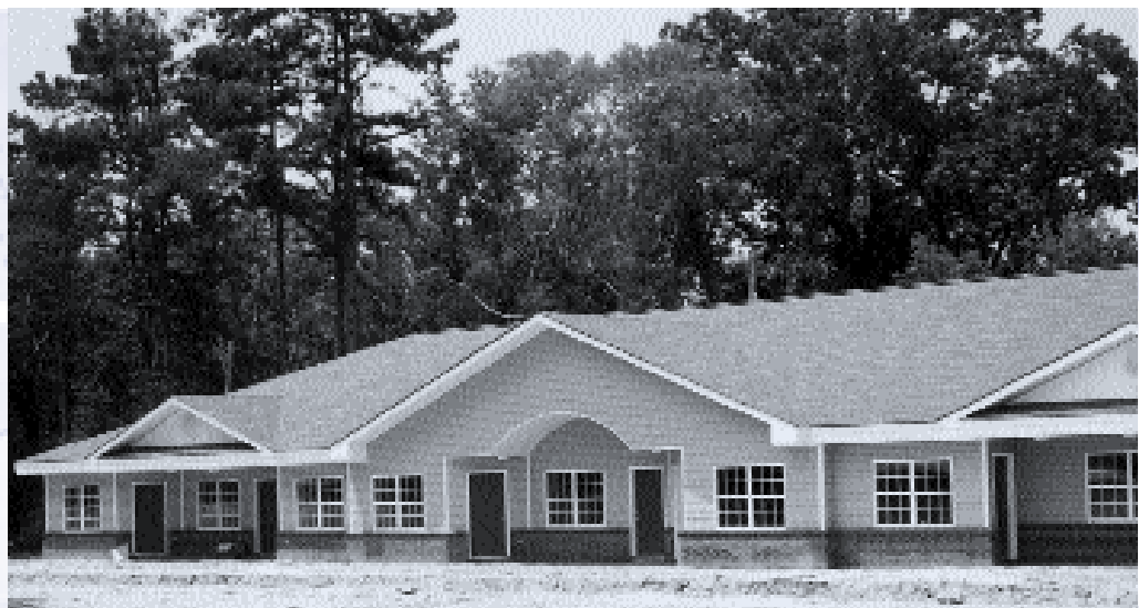
Exterior Solutions is the general contractor for this 9-unit senior housing development in Chidester, Arkansas.
