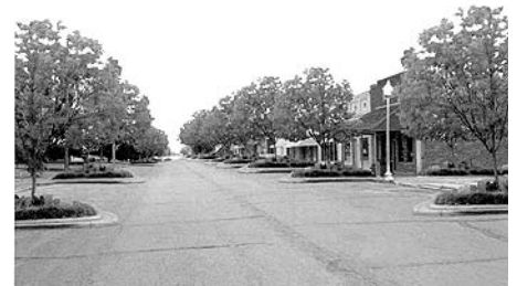
Using a $44,000 donation from Southern, Drew is making Main Street more vibrant and pedestrian friendly through a streetscape project.
