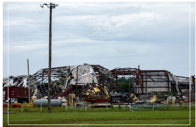
Structural tornado damage in Trumann, Ark.
